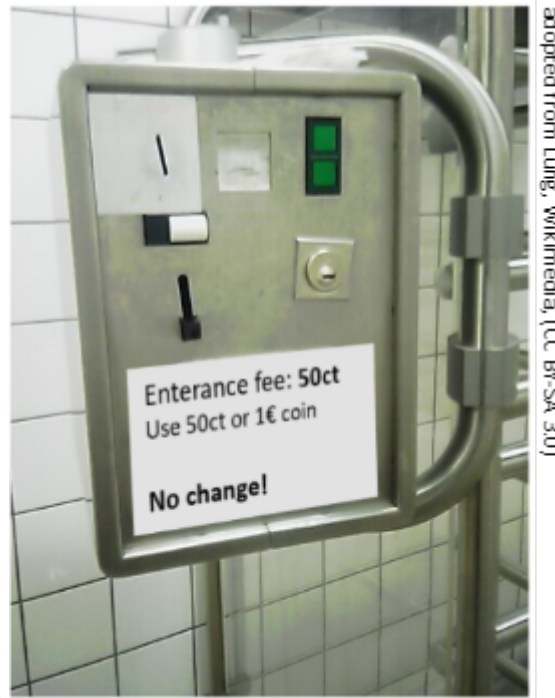
Fig. 11: Entrance Control for Toilets
